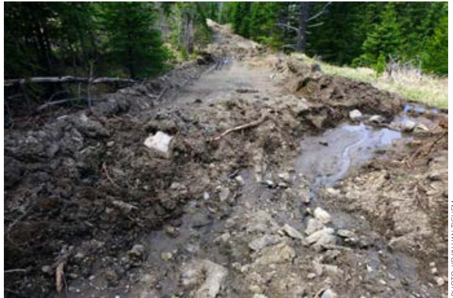
Groundwater escaping from one of many road cuts in the upper Oldman River basin
