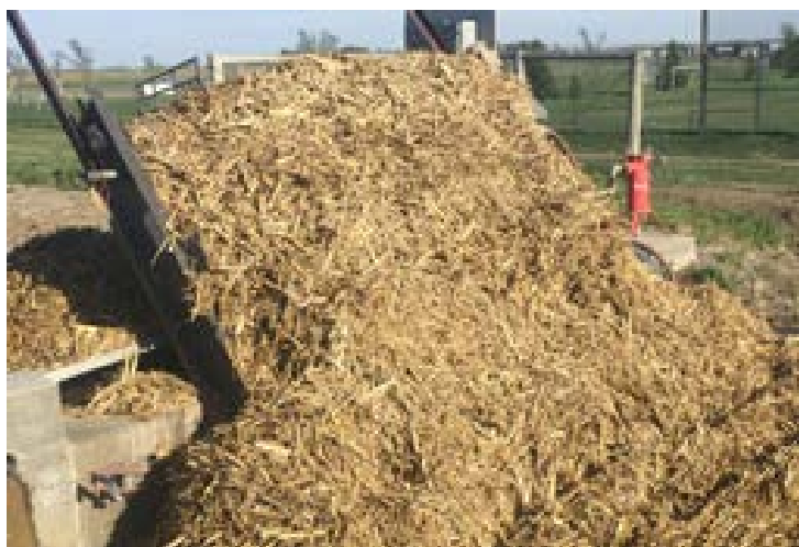
Soil isn’t the only thing that blows around in those storms. This is a canal trash rack from spring 2021 clogged with blown crop residue. We don’t typically think of irrigation districts as neighbours either, but in this case, they are. PHOTO: SMRID
