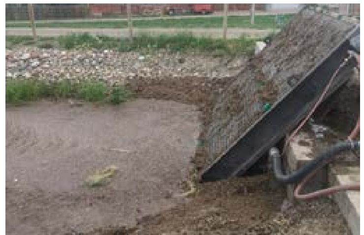
SMRID saw debris blown into canals at a rate to clog trash racks. PHOTO: SMRID
