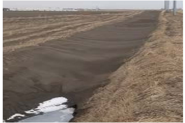
Blow-dirt clogged canal. PHOTO: KEN COLES
